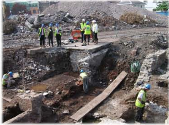
excavation of lift shaft next to Trench 3
