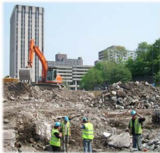
excavation of Trench 2 gets underway
